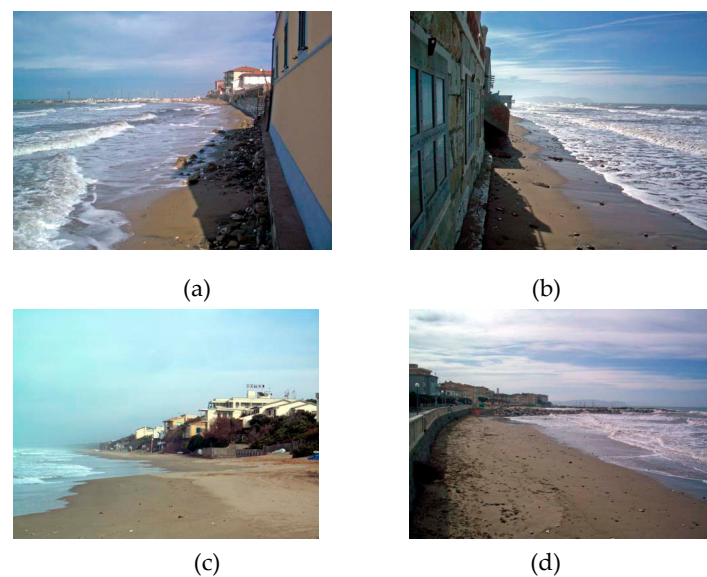
Figure 4. San Vincenzo shore at the start of reshaping works on the harbor (04/03/2006). (a,b) South harbor area; (c,d) North harbor area [40].
