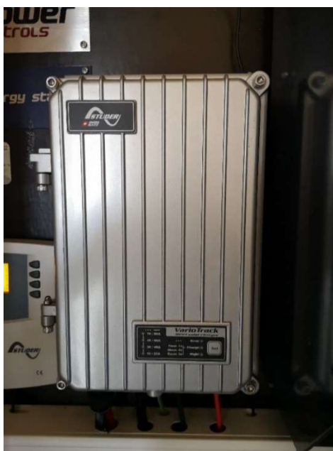
Figura 3.8 Studer Variotrack /Regulador
