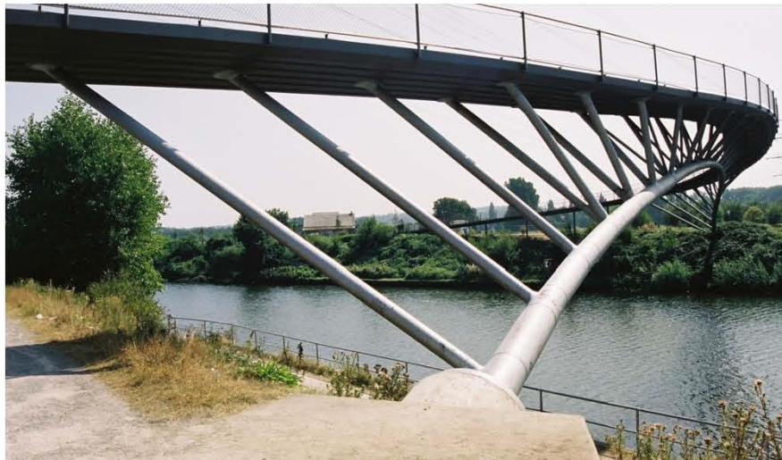
Figure 4. Ripshorst footbridge (Photo courtesy of Nicholas Janberg, structurae.net ).
