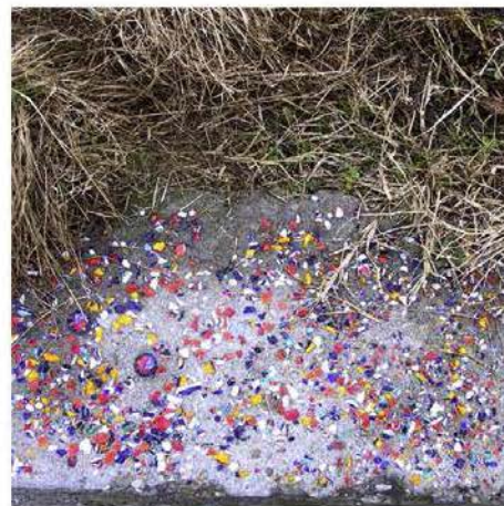
[24] THE PAVING ALONG THE MARGIN OF THE CLOSED WATERWAY OF SACCA SERENELLA, MURANO, REALIZED WITH CONCRETE MIXED WITH RESIDUE FROM THE PRODUCTION OF GLASS. PHOTOGRAPH BY IUAV STUDIES & PROJECTS, 2002.
