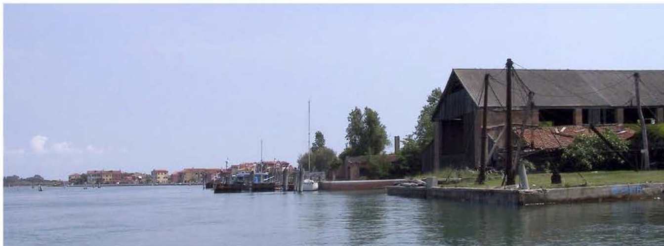
[10] RIO DI SAN GIULIANO, WAREHOUSES BUILT IN PART ON THE MAINLAND, IN PART OVER THE WATER USING A PILE SYSTEM. PHOTOGRAPH BY IUAV STUDIES & PROJECTS, 2002.
