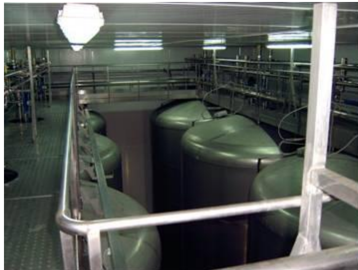
Figure 1 Bulk storage aseptic tanks (Photo by A. López-Gómez).
