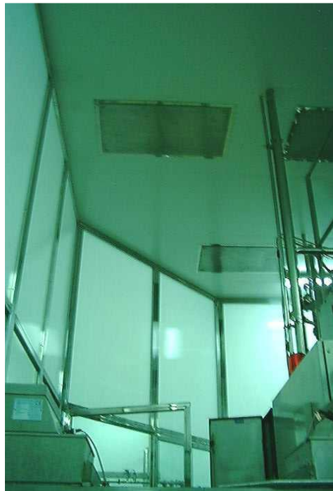
Figure 3 Class 10.000 clean room as a closing of a Class 100 clean room, for ultra-clean packaging of fruit juices (Photo by A. López-Gómez).
