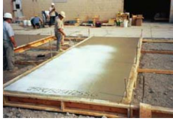
Figure 42: Polymeric curing membrane application
