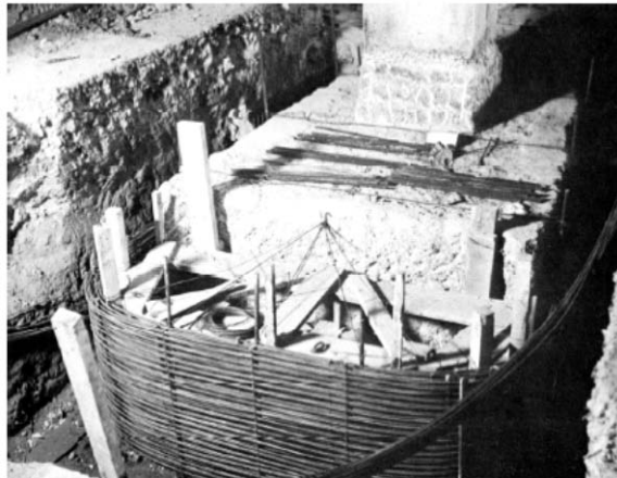
Figure 2.7 Horizontal prestressing on footings in Le Havre
