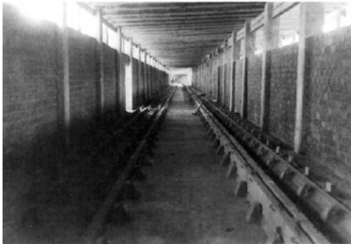
Figure 2.8 First casting bed for precast/prestressed members
