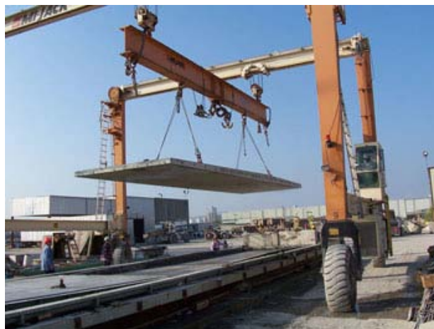
Figure 3.21 Gantry crane lifting a panel
