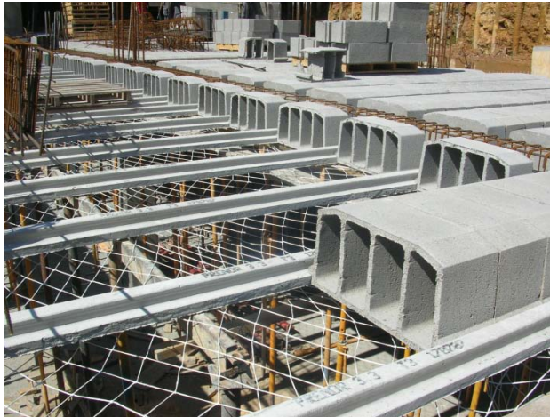
Figure 4.3 Semi-resistant joists slab with safety net and propping
