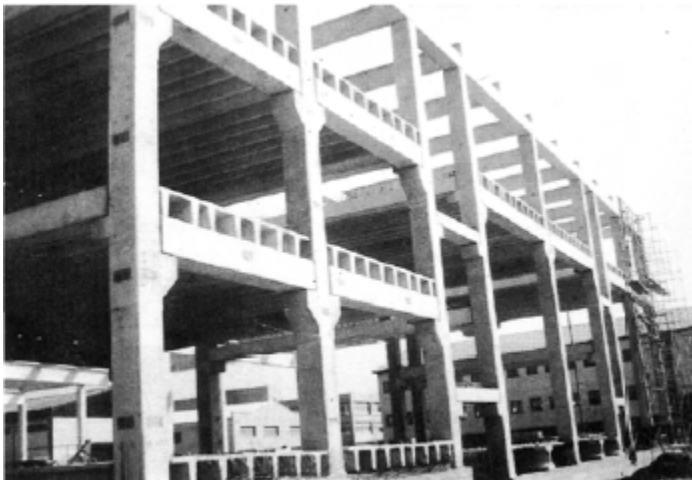
Figure 2.9 Double-t beams slab in the 1970's
