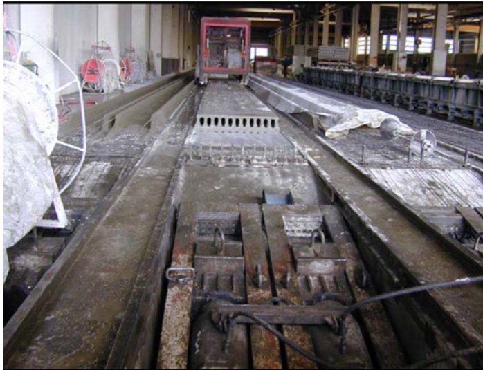
Figure 3.3 Long-line production of pre-tensioned members (Prefabricados Castelo).
