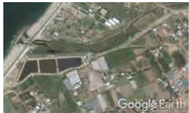
Figure 2.2.2.1 Wadi Gaza wetland (lower end of the Wadi) and temporary wastewater plant in the left of the photograph.
