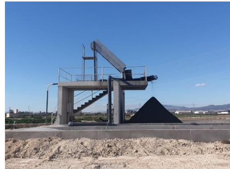
Photo 4. Worm screw separator
