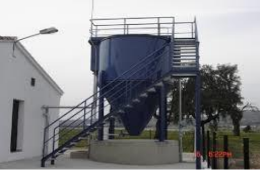
Image 6. Vertical static decanter
