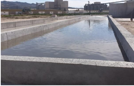
Image 5. Horizontal static decanter
