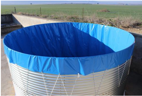
Image 2. Slurry storage tank
