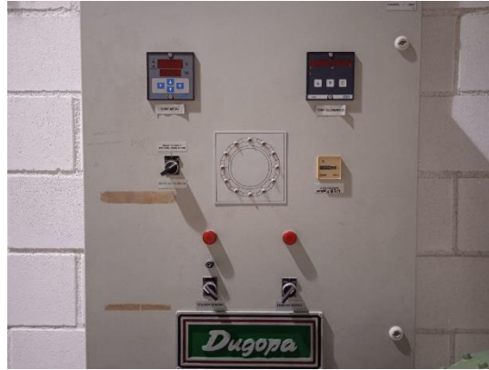
Figura 3.5 Panel de control del horno
