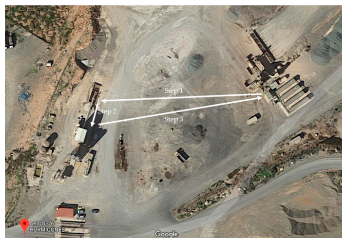
Figure 12. Path used by the drone to execute the mission in a concrete plant.
