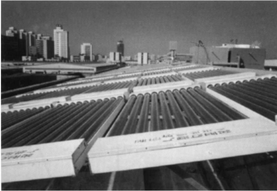
Fig. 1. View of the integrated solar cooling and hot water system at Shenzhen.
