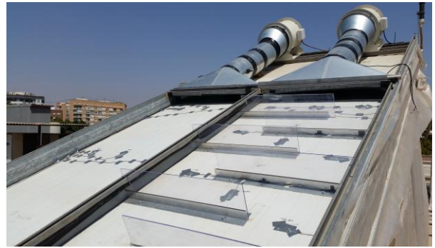
Fig. 2. View of the inside of the ducts. Setting A (Left). Setting B (Right).
