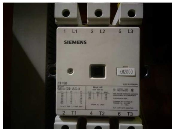
Figura 3-32: Contactor del regulador principal
