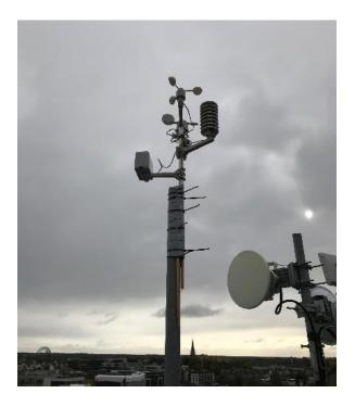
Figure III.17. A weather station installed on the roof of Østfold University College.
