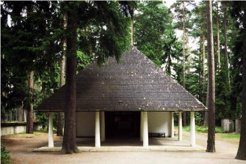
[14] ASPLUND. WOODLAND CHAPEL. ENTRANCE FAÇADE.
