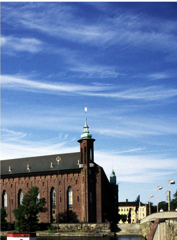
[3] ÖSTBERG. STOCKHOLM CITY HALL. EAST FAÇADE.
