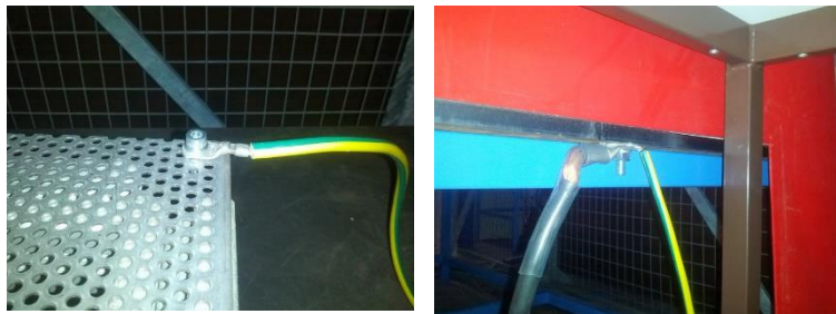
Fig. 65. - a,b Welding Ground Connection
