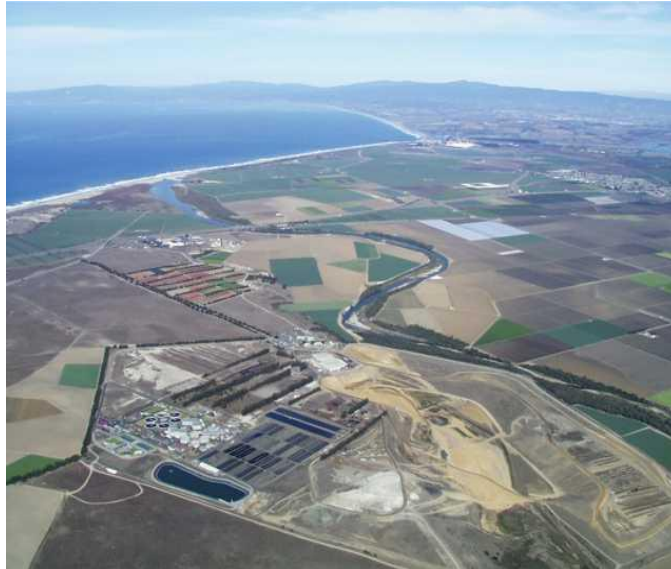
Picture 3: Aerial view of the experimental farms and the wastewater treatment plant “WWTP”, where the Monterrey Wastewater Reclamation Study for Agriculture was developed.
