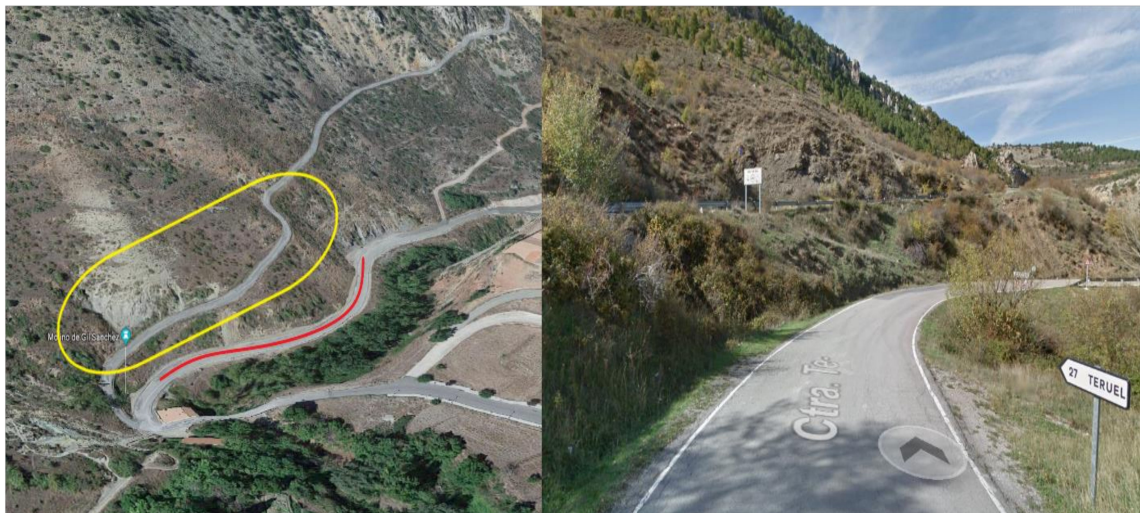
Figure 8. Location of the road to be extended (red) and existing road to be maintained (yellow).
