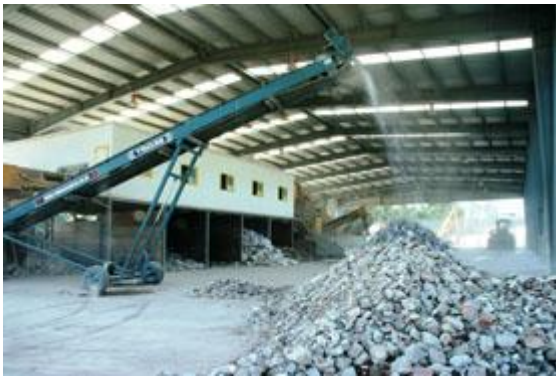
Figure 9. Mobile crusher with electromagnet
