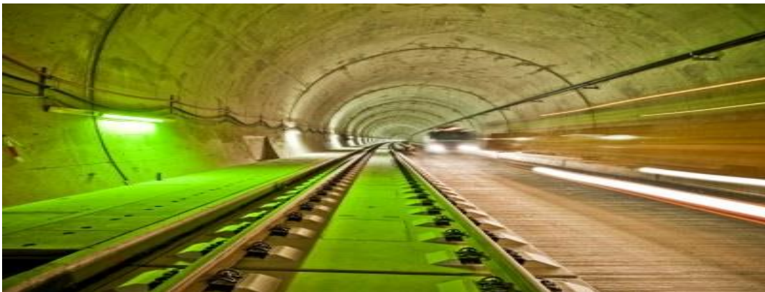
Figure 2. BBT railroad tunnel
