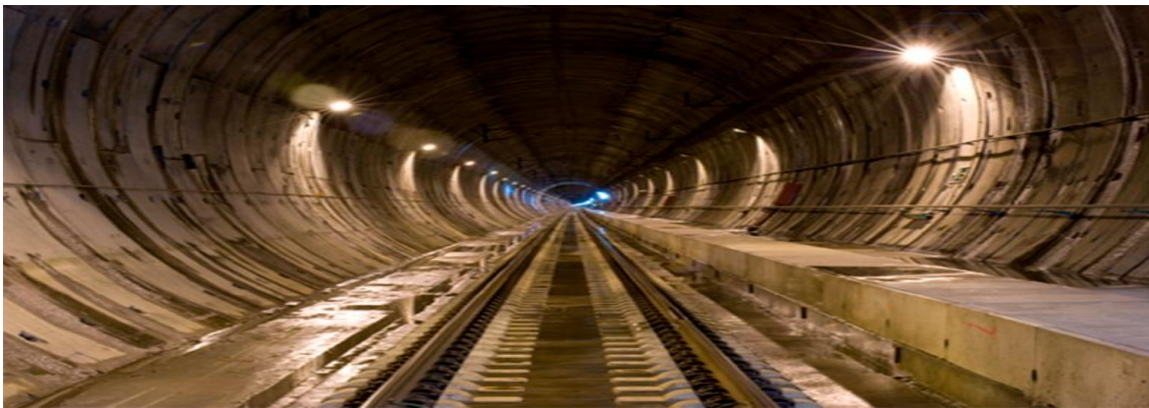
Figure 1. Guadarrama railroad tunnel
