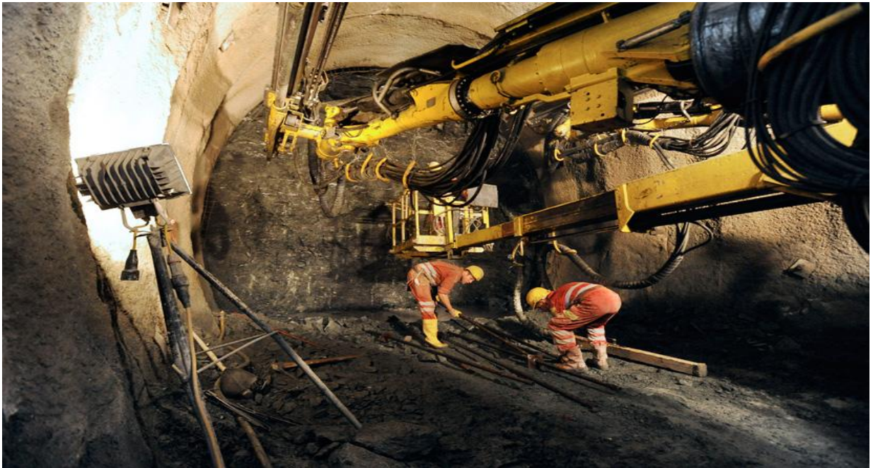
Figure 22. Drill and blast excavation machine
