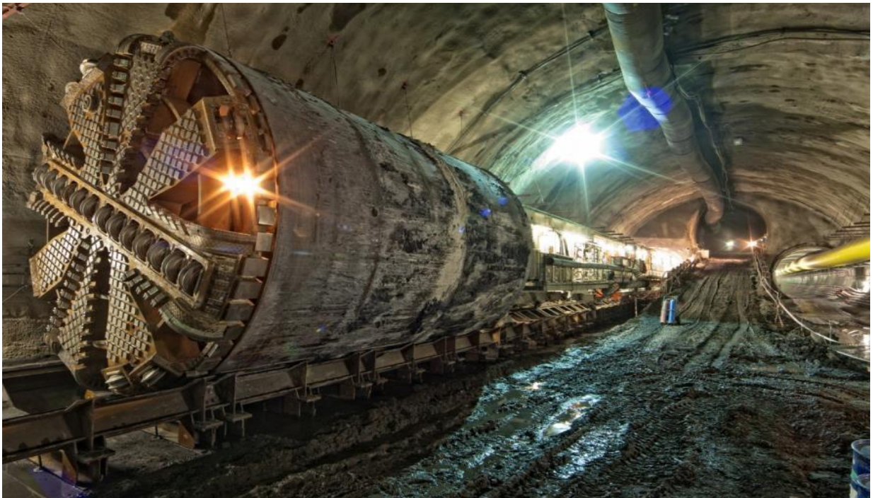
Figure 20. TBM Brenner Base Tunnel
