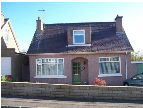
Figure 3.1. Front facade of the property.
