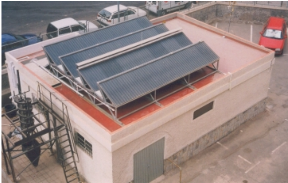
Solar roof erected at the Scholl of Engineers in the Polytechnic University of Cartagena (Spain)
