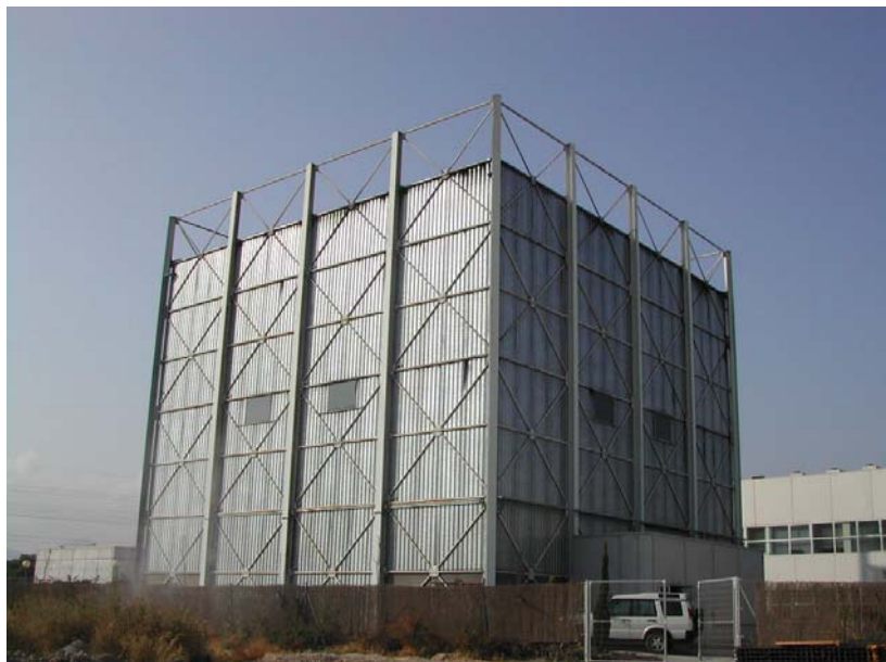
Fig. 1. The “Fire Atrium” of the Technological Metal Centre, Murcia, Spain.
