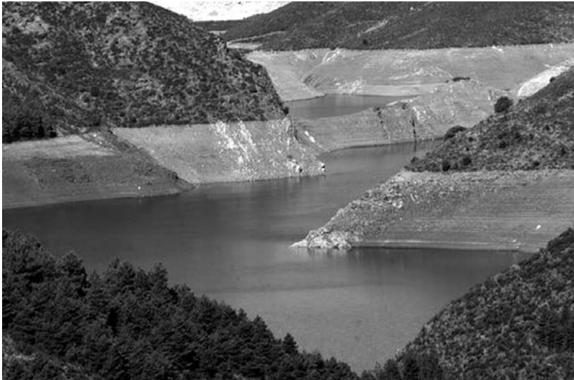
FIG. [1] DAM OF EL ATAZAR, SPAIN, 2005. FIG. [2] DAM OF AGUIEIRA, PORTUGAL, 2011.
