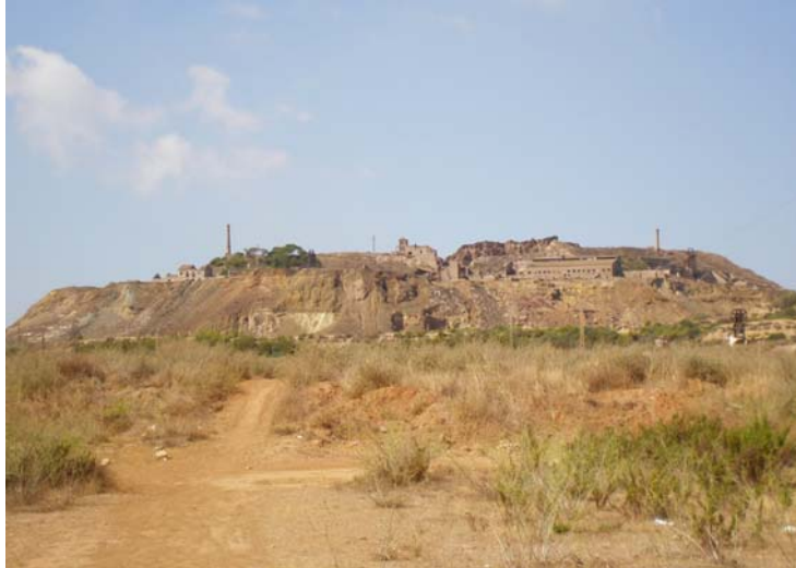
Figure 6: View of the Cabezo Rajao, mountain exploited from Roman epoch that take his name for the great gap that stayed in it after the extraction of the vein of galena that was finding in his interior. We Can appreciate also mining elements as chimneys and head frames. In all this space we try to place a Thematic Museum of the mining industry.
