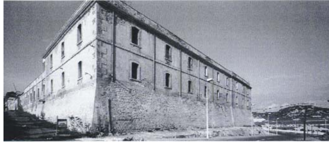
Fig. 2. University building to be rehabilitated
