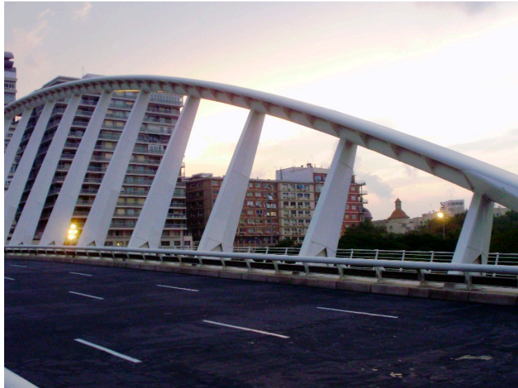
Figure 6. La Alameda bridge. (See Tzonis [17], Jorquera-Lucerga [18] and Jodidio [19]). Photo: J.J. Jorquera-Lucerga.
