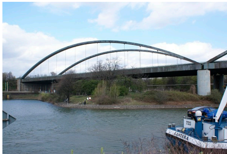
Figure 2. Bridge for the Autobahn A-42. Rhine–Herne Canal. Photo: N. Janberg (reproduced with permission from Structurae [7], 2008).
