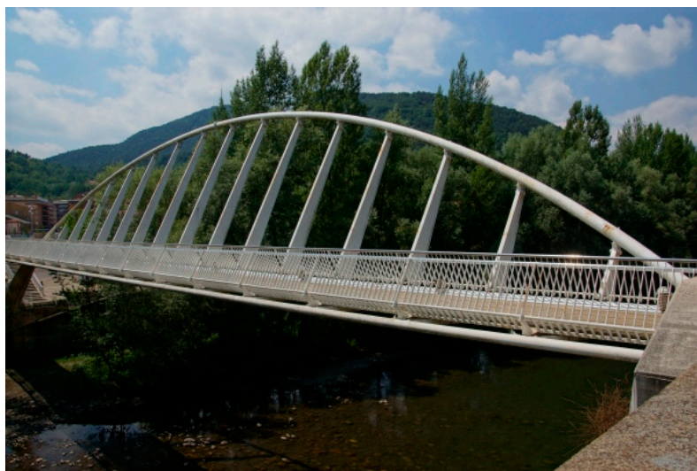
Figure 5. La Devesa footbridge (See Tzonis ([17] and Jorquera-Lucerga [18]) Photo: N, Janberg (reproduced with permission from Structurae [7], 2011).
