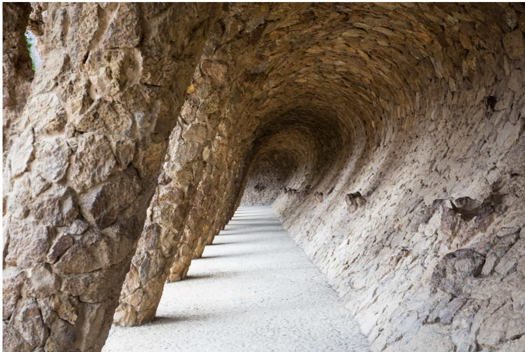
Figure 1: Retaining walls of the Güell Park at Barcelona
