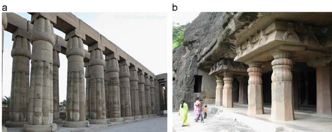
Figure 27: a) Ancient Egyptian columns inspired by a bundle of papyrus plants in Luxor Temples, Egypt, built in 1400 BC; b) ancient rock-cut columns with lotus capitals in Ajanata caves in India build in 200 BC.
