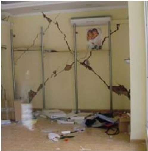
Figure 35 Damage interior walls. Lorca Earthquake 2011 (Tomas Espin, 2011)
