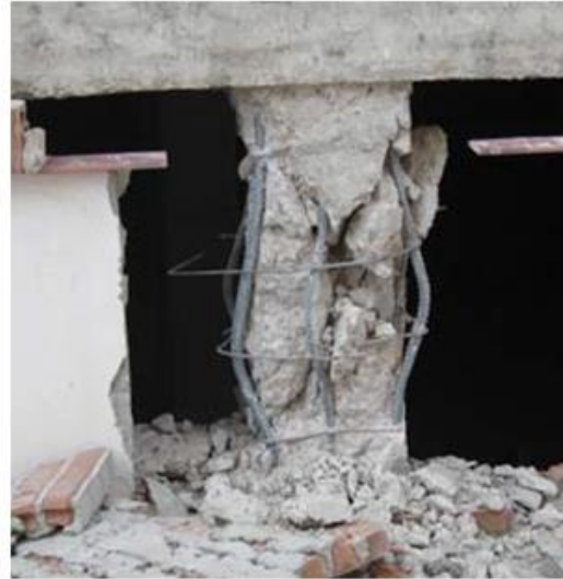
Figure 28 short pillars in Lorca earthquake 2011 (Tomas Espín, 2011)
