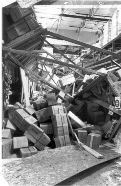
Figure 40 Damage to overloaded racks during the 1994 magnitude-6.7 Northridge Earthquake (FEMA 460, 2005).
