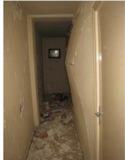
Figure 35 Damage interior walls. Lorca Earthquake 2011 (Tomas Espin, 2011)
