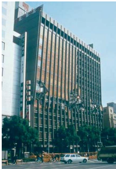
Figure 21 upper storey failed (Hugo Bachmann, 2003)
