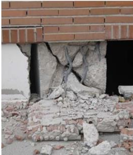
Figure 28 short pillars in Lorca earthquake 2011 (Tomas Espín, 2011)
