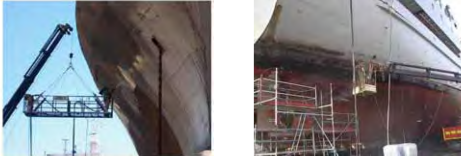
Figure 1. Present method for hull blasting: a dangerous manual task
